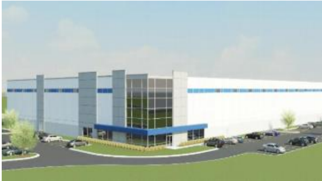
First Joliet Logistic Center
