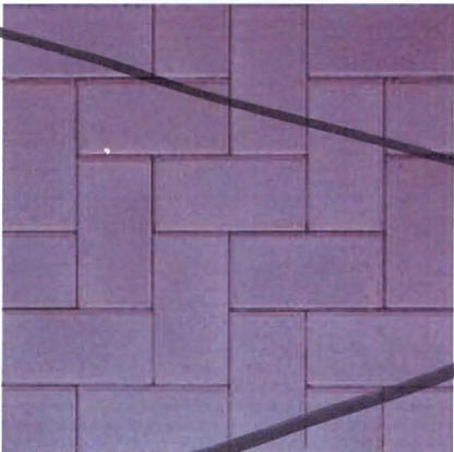
Pavers Exterior Accent Surface
