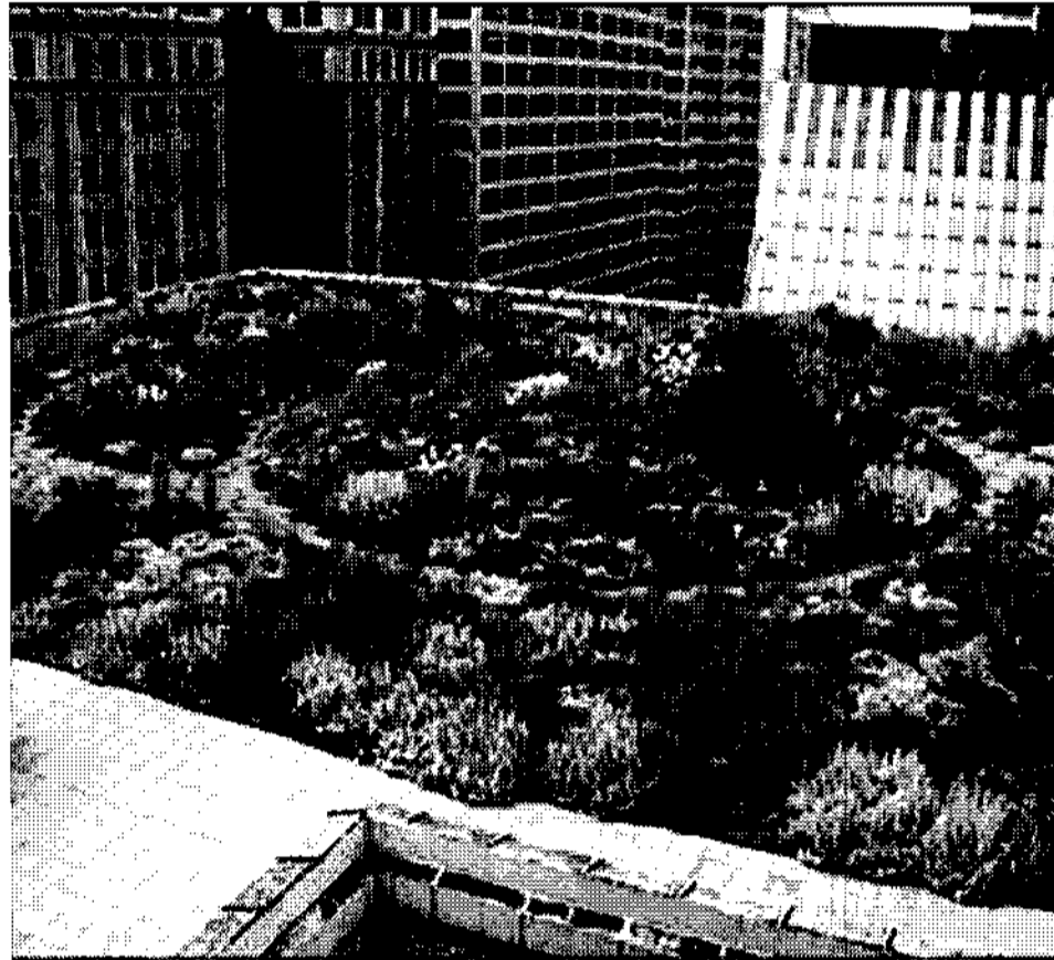
7 EXAMPLE OF GREEN ROOF SCALE: N/A
