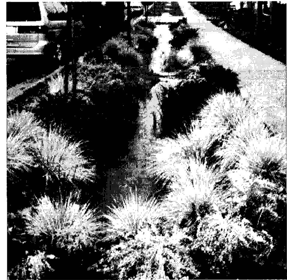
4 EXAMPLE OF BIOSWALE SCALE: N/A
